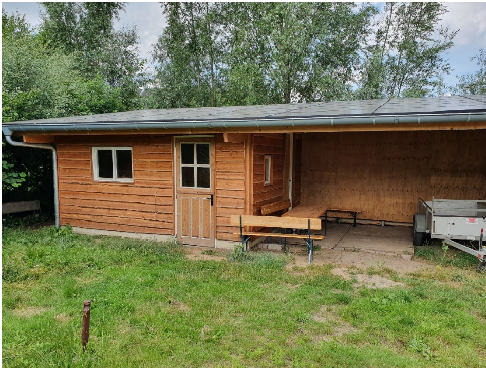
Figure 24. Solar carpark shed
