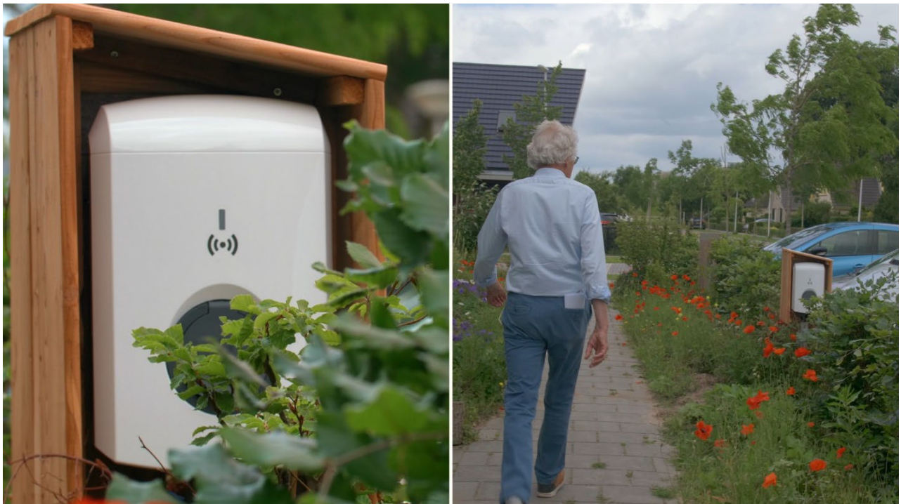
Figure 21. Alfen pro EV charger in Vriendenerf charging inhabitant’s EV by solar power
