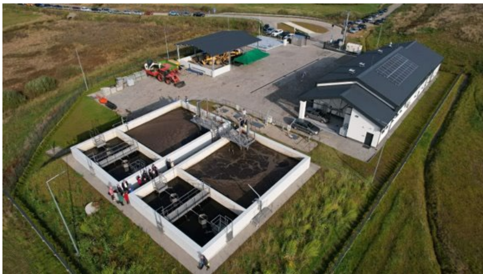
Figure 15: Sewage treatment plant in Przywidz
